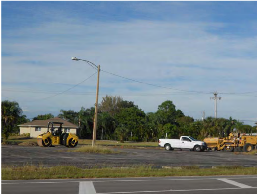
VIEW OF NON-CONTIGUOUS FORMER PARKING LOT ON PALM TREE BOULEVARD
